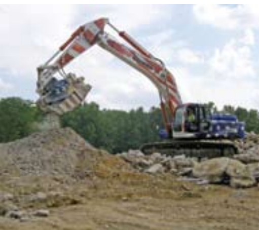
Works have already begun on the massive housing project.
