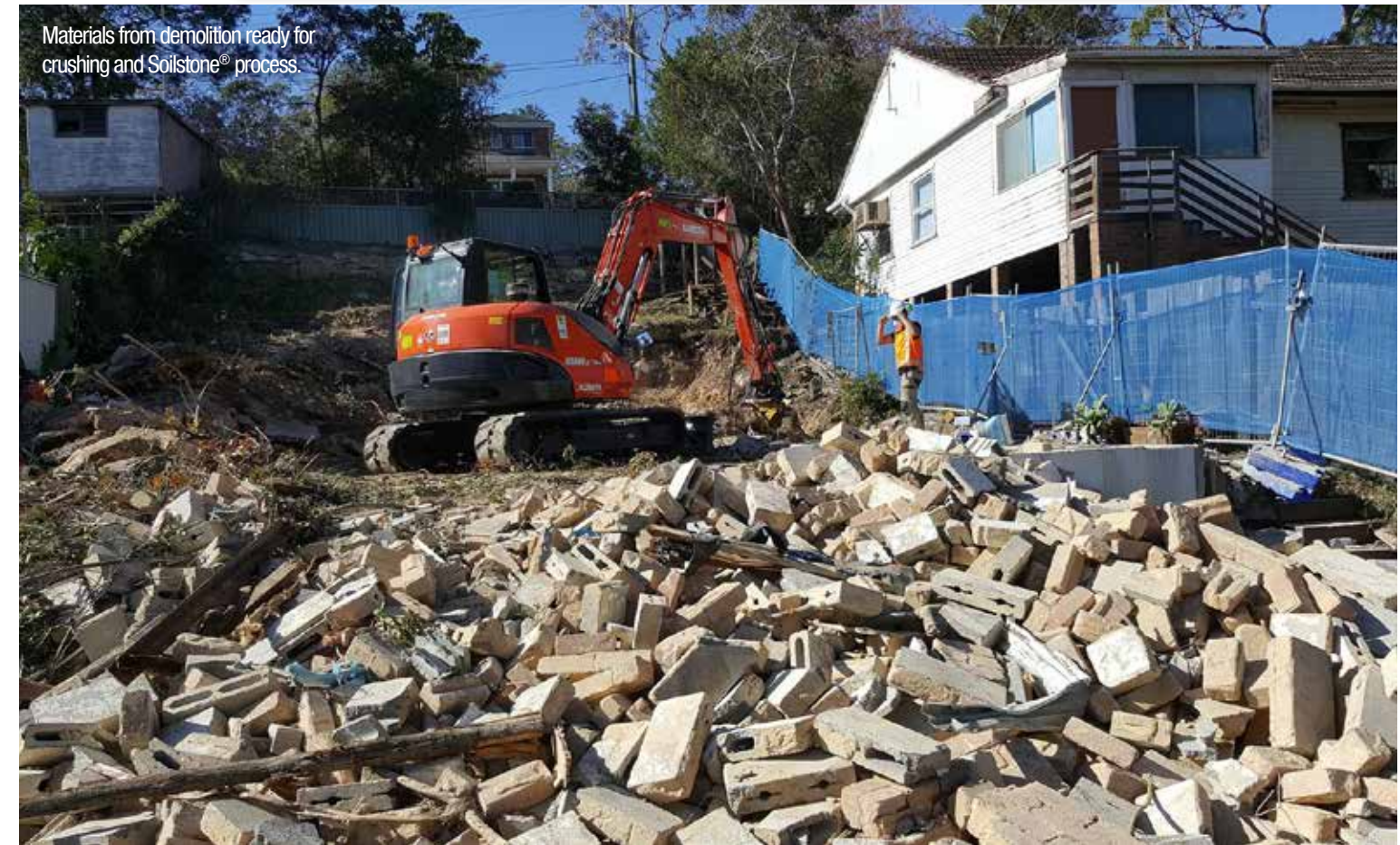
The MB Crusher bucket crushes demolition material.
