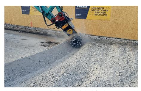
Above: ERA has used MB Crusher drum cutters to help with demolition works on an old bridge in Berlin. Here is one of the models chosen for the project, the MB-R900.
