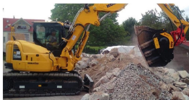
■ MB's BF60.1 can recycle building materials on site.
