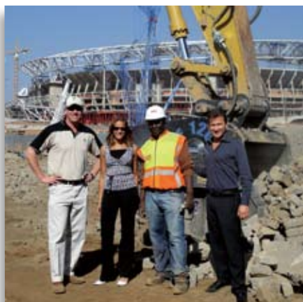
MB's crusher bucket is being used to clear inert material at the new Soccer City Stadium.
