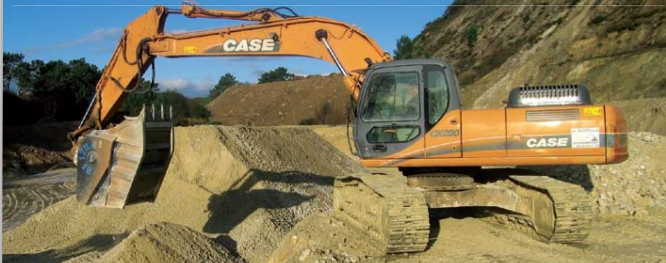
A MB BF120.4 bucket crusher on a Case CX290 excavator.
