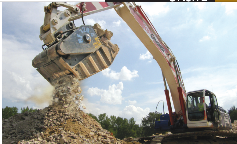
An MB crusher bucket at work on the US development
