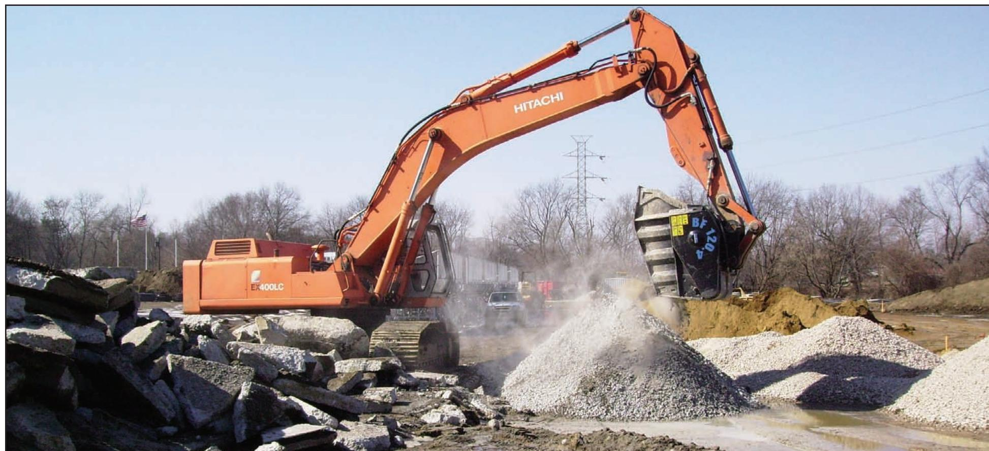
The Eco-Crusher creates revenue by turning useless debris into material that can be used on site or on other jobs and charged for — or sold to other contractors.
