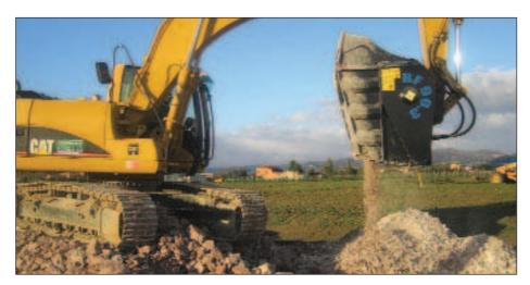
The company demolished one whole bridge span and crushed the material on site using a Caterpillar 325 LN excavator and an MB crusher bucket. Thanks to its 3m width, the slightly oversized machine guaranteed the stability needed to carry out the crushing.
