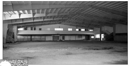
In Culver City, Calif., the project involved removing a 5in. (12.7 cm) thick concrete slab from a former roller skating rink.
