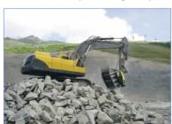
ing the material and producing the stabilized pavement directly on site, thereby saving time and reducing costs. Tokyo has one of the most expensive transportation systems in the world, and trucks are forced to make many trips to complete a job. One problem that MB effectively solves since materials are crushed on site and consequently there is no need to transport them to another location.
